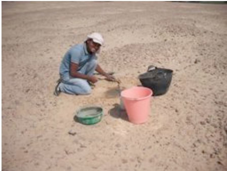
Fig.4: Kamal Helmy Quftawi cementing in ST16, one of the new iron control points.
